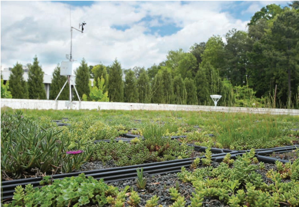
The green roof of the Learning Center consists of three types of sedum and one ice plant that each bloom multiple times per year. The weather station is connected to the BAS and measures min./max. dry bulb air temp, RH, dew point, solar radiation, hours of sun, net radiation, barometric pressure, min./max. wind speed, wind direction, gusts, gust directions, and CO 2 .
