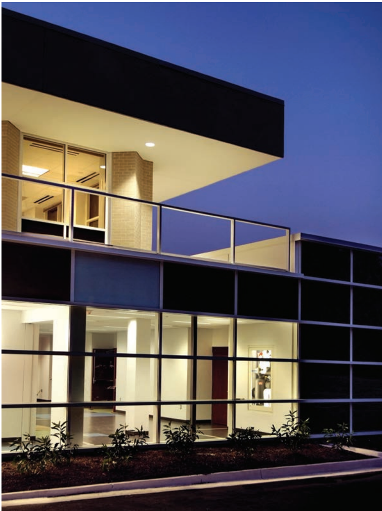
Photocells, occupancy sensors, and occupancy schedule are used to control lighting use. A change-out to LED lights in some locations is being considered.
